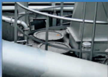
Optimum protection for storage silos and elevators: the EGV explosion vent.
