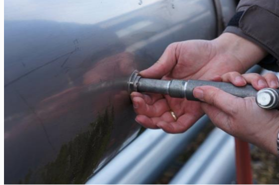
Installation of adapter
